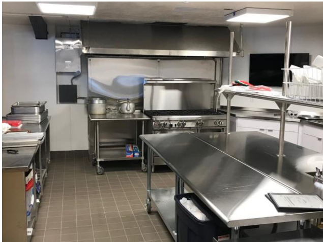
New flooring, stove, and stainless steel all around.
